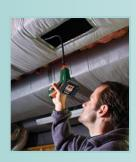
Extech Borescope features a 2.25" color monitor with video output for viewing on any monitor and a waterproof 9mm camera with bright LED lights.
