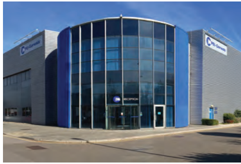
European Headquarters & Production Facility, Southampton, UK
