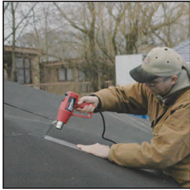
Weld Roofing Membrane
