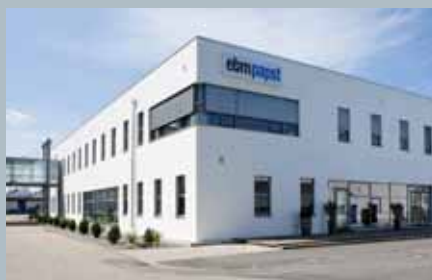
Left: Our headquarters in Mulfingen Right: Our location in Landshut
