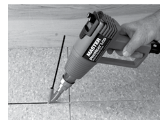
Welding Flooring Material
