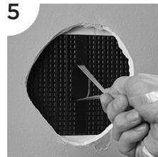
Carefully center back plate in damaged area so adhesive tape makes contact with paper on the backside of wall. Pull strap to secure tape to wall and hold for 30 seconds using moderate pressure, DO NOT over pull strap.
