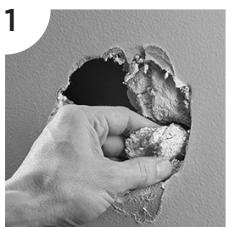
Clean damaged area by removing all dust and loose debris on both inside and outside wall. Tape on back plate requires a dust free surface for best adhesion.
