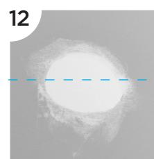
Apply a primer/sealer and paint according to the manufacturer's instructions. If necessary, additional coats of compound can be applied before or after priming.
