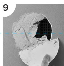
Use putty knife to slightly overfill damaged area with wall repair compound - overfill allows for flat sanding of the repair when dry.
