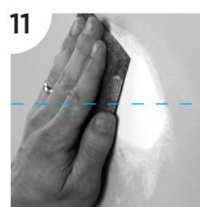
Once surface is completely dry, sand flat to finish. Repair should be allowed to dry overnight.
