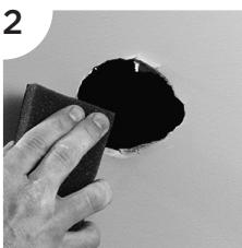
Thoroughly sand outside edge of hole, making sure surface is as smooth as possible. All edges of the paper should be recessed below the topside wall.
