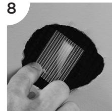
Lightly apply supplied tape over center hole. Trim if necessary.
