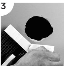
Remove the white backing from both strips of double-sided tape.
