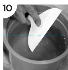
After damaged area is completely filled with wall repair compound - overfill allows for EACH STROKE and slowly smooth compound using a VERY LOW angle.
