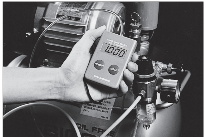
▲ Measurement of source pressure from a compressor.
