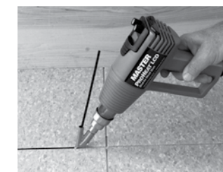
Welding Flooring Material
